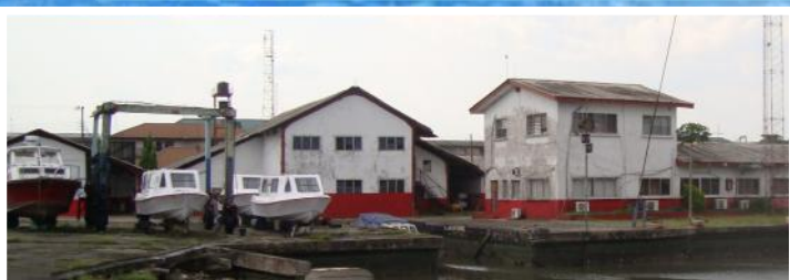
Slipway & Jetty Services
